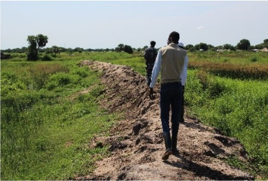
Photo 13: Earthen dyke, northern Bor
