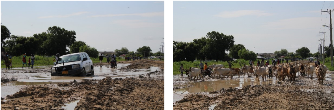
Photo 3: Vehicle and cattle having problems navigating poorly drained muddy road
