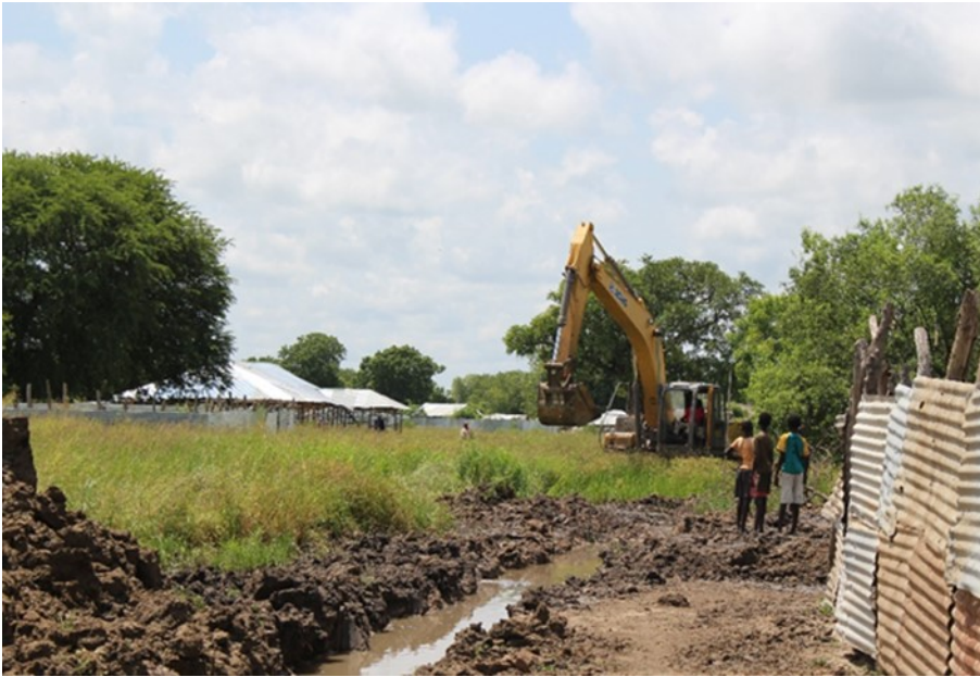
Photo 11: Excavator at work in Bor, digging emergency drains
