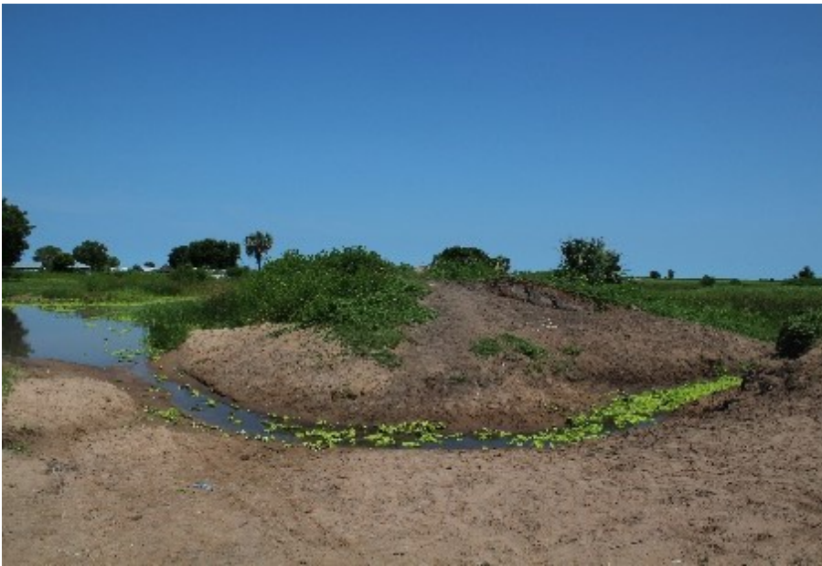
Photo 15: Man-made breach in Nile dyke to allow discharge of urban (rain) water
