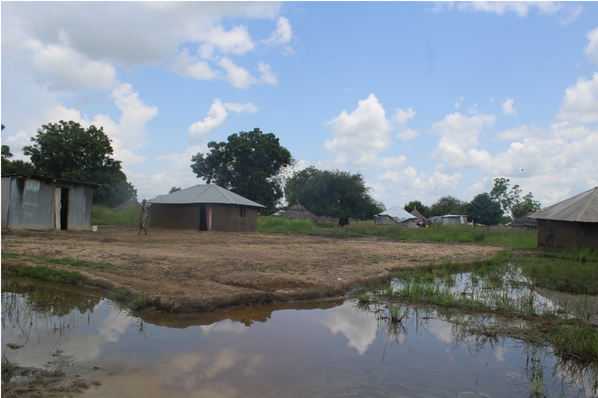
Photo 2: Homestead dyke in Bor town
